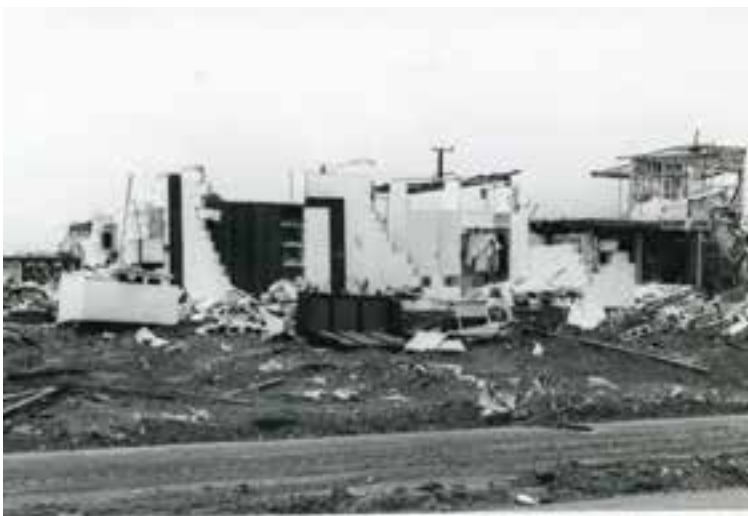
Demolished house in Bell St Nakara. 4 People died when wall collapsed.
