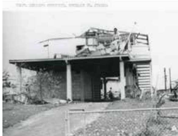
Const Herald's Residence, Rothdale Rd Jingili.
