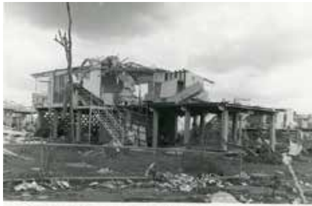
Constable Kennedy's Residence. Rothdale Rd Jingili
